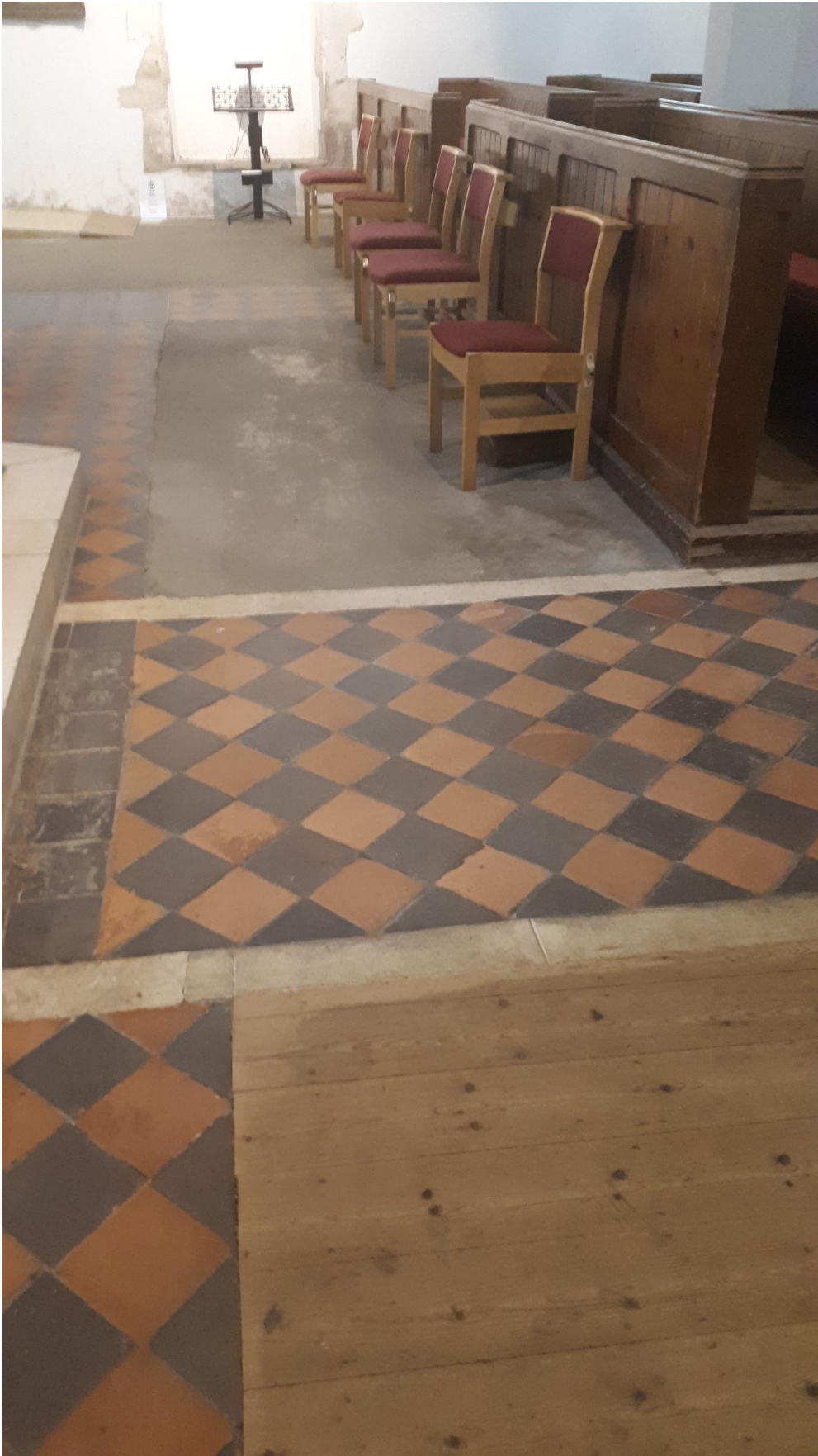
Floor at the front of the nave showing the mix of pine, Victorian tiles and concrete
