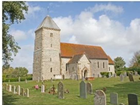
View from the south-west corner of the churchyard
